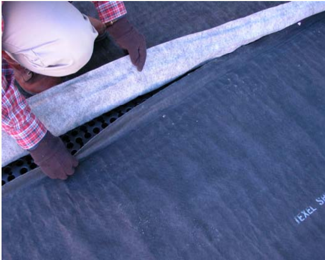
Overlaps drain core at seams
