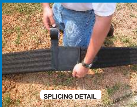
INSTALL AND TAPE FITTINGS
